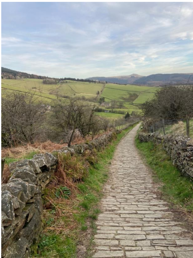
Stone flags used on Saddlers Way, Macclesfield Forest (bridleway)
